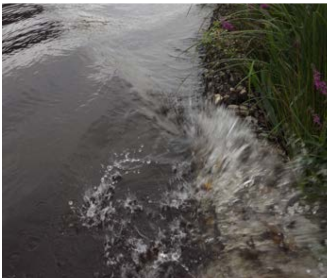
Pre-filled Rock Rolls dissipating wave energy
