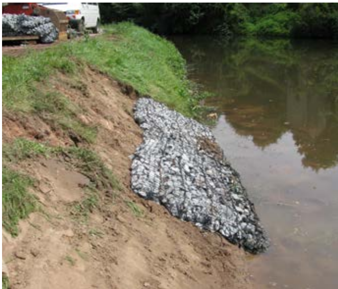
Pre-filled Rock Mattress installation before and after
